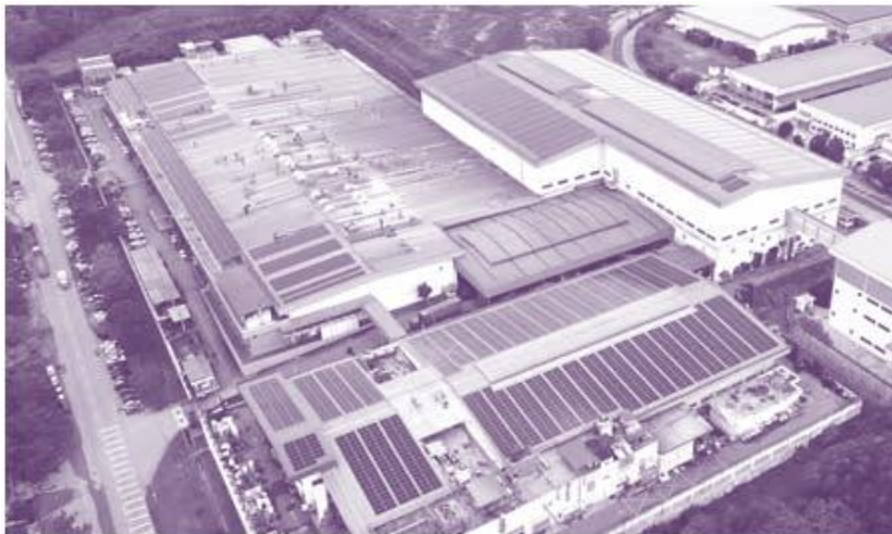
2,494kWp and 832.88kWp rooftop solar system at our plants in Nilai, Negeri Sembilan
