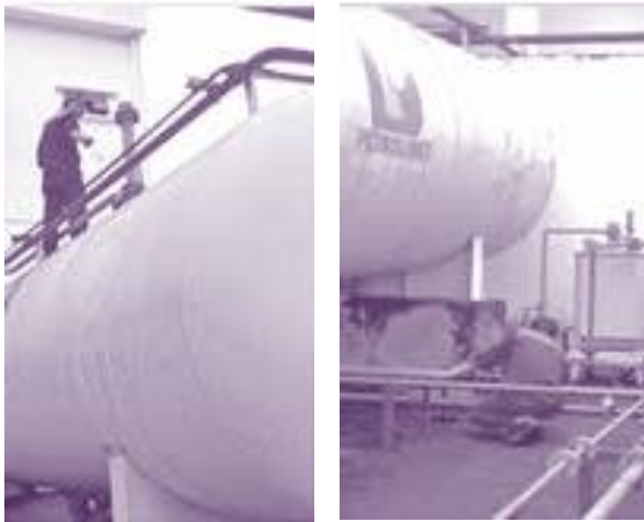
LPG Station safety check – Kian Joo Can (Vietnam) Co., Ltd.
