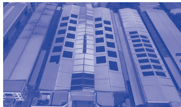
456 kWp solar system at Aik Joo Can Factory Sdn. Berhad Lot 2211
